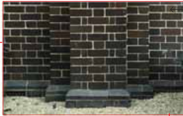
REFERENCE IMAGE. EXISTING BRICK PIER ELEVATION
